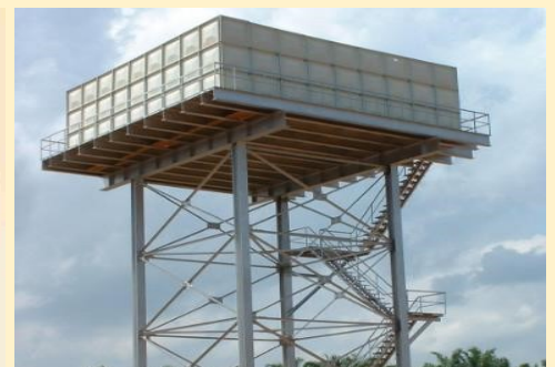
Elevated water tank
