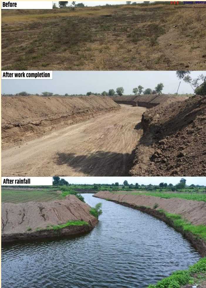
Diversion channel constructed to direct water to storage areas
